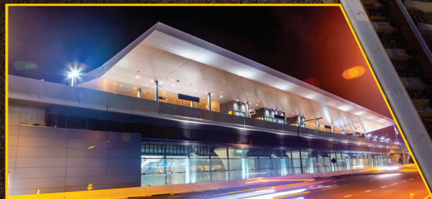
DULLES CORRIDOR METRORAIL
