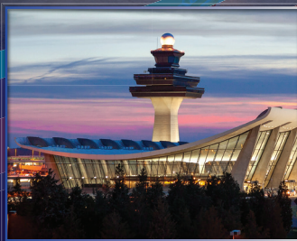
DULLES INTERNATIONAL AIRPORT
