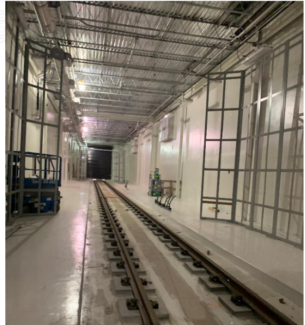
Inside Train Wash Facility
