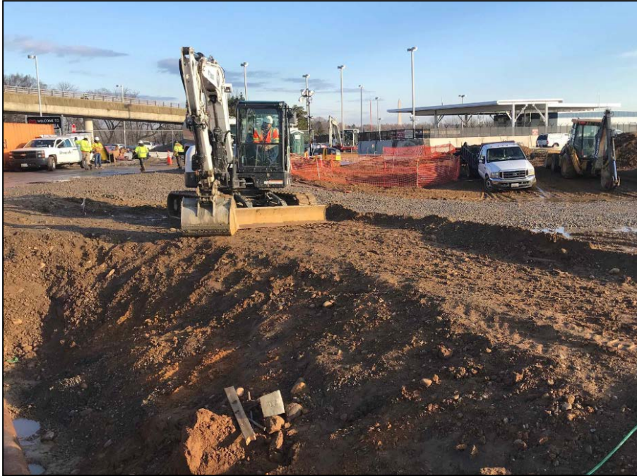
Blast Wall Foundation Excavation Completion: April 2019
