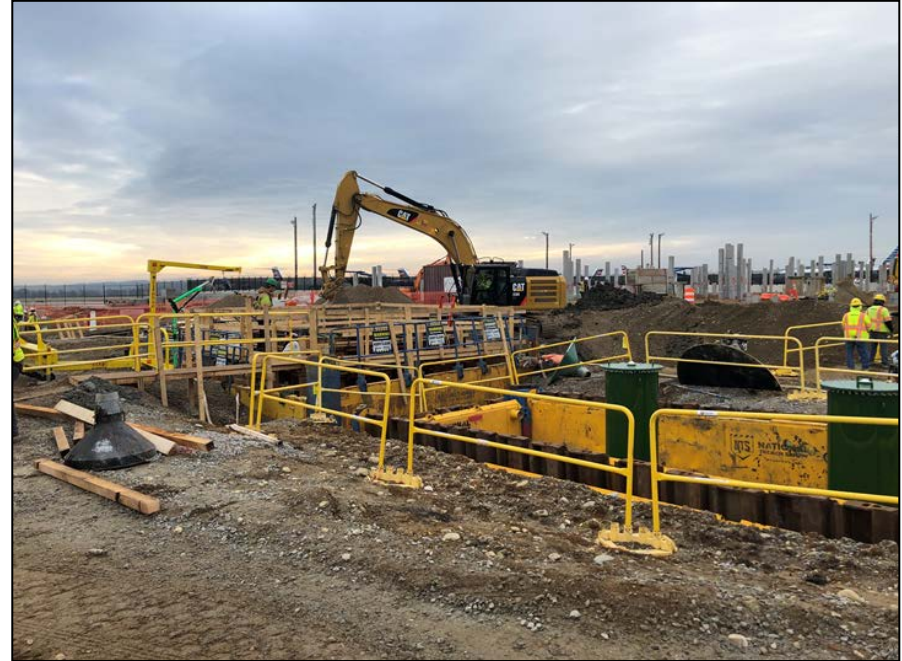
Oil/Water Separate & Glycol Collection Completion: March 2019
