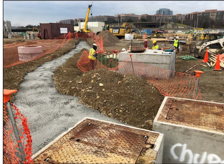
Electrical/Comm Duct Bank Installation Completion: March 2019
