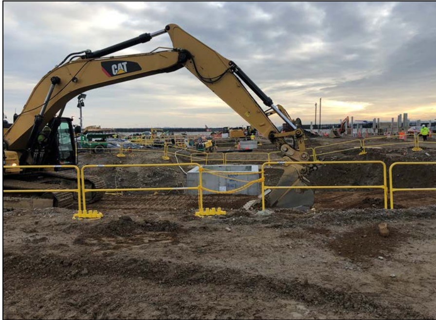
Storm Sewer Installation Completion: March 2019
