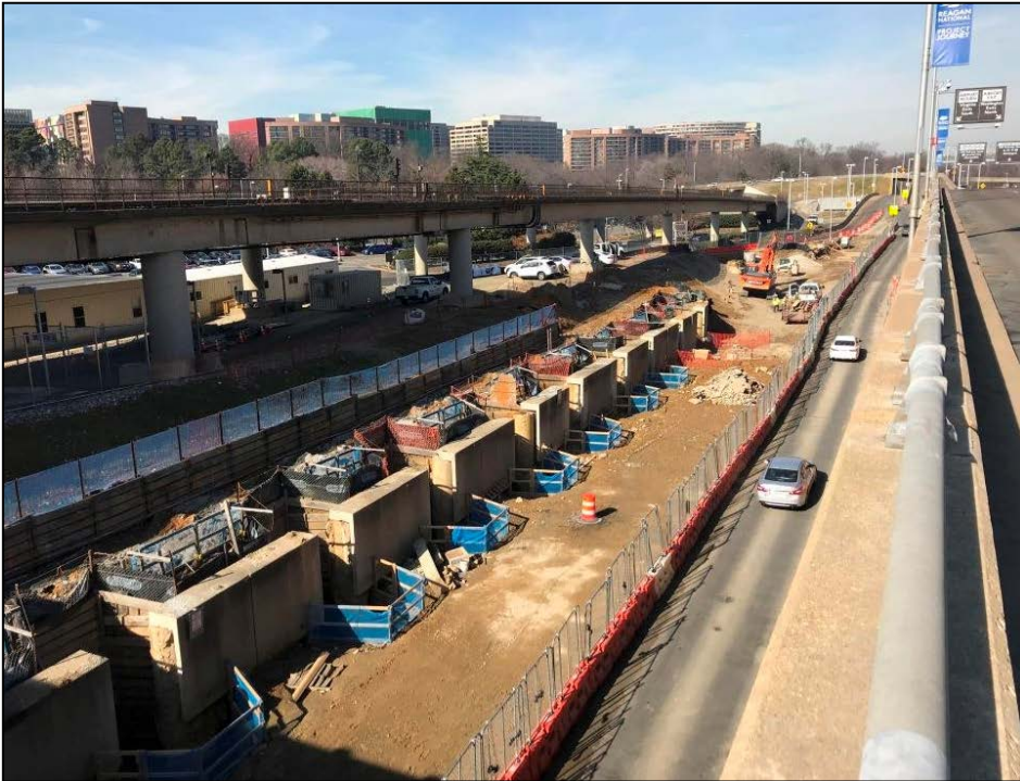
Excavate & Install Box Culvert Completion: March 2019
