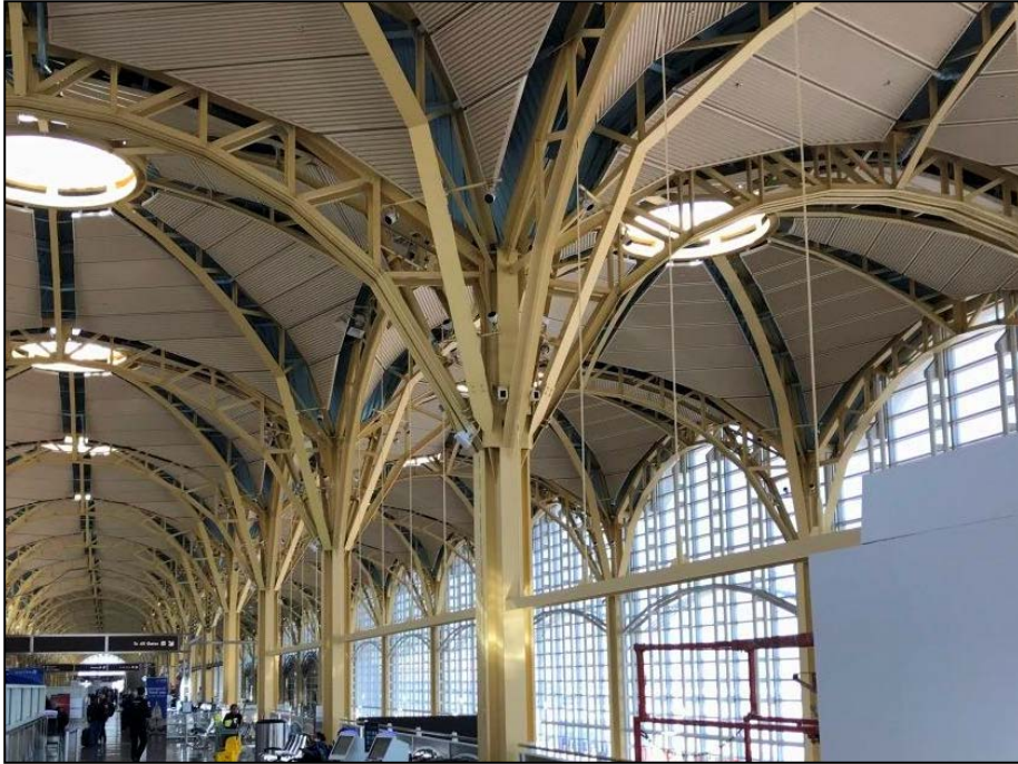
Security Identification Display Area (SIDA) Wall Completion: June 2020
