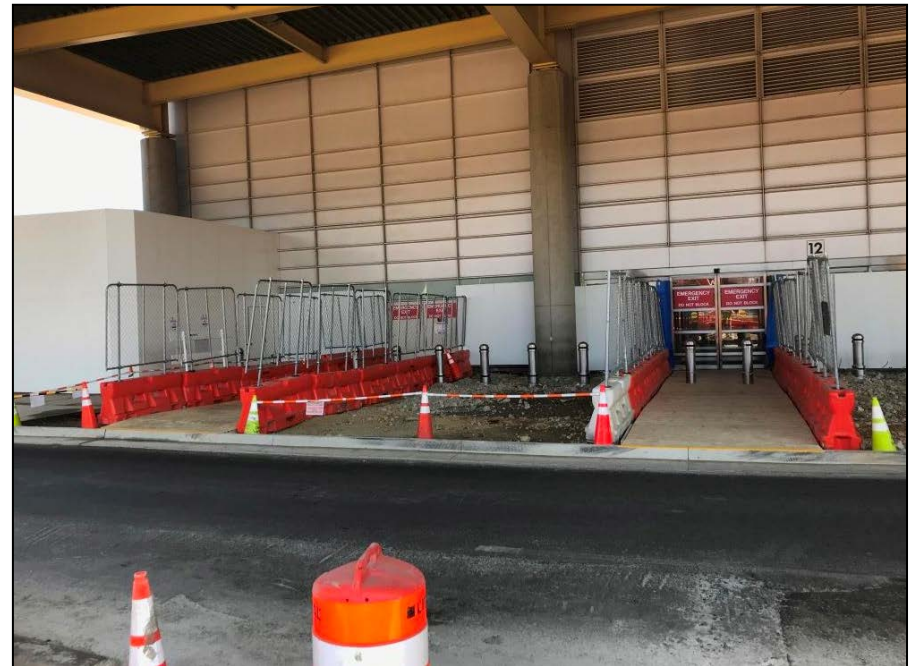
North Door Emergency Egress Completion: March 2019
