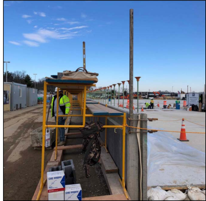
Blast Wall – Concrete Block Scaffolding Completion: April 2019
