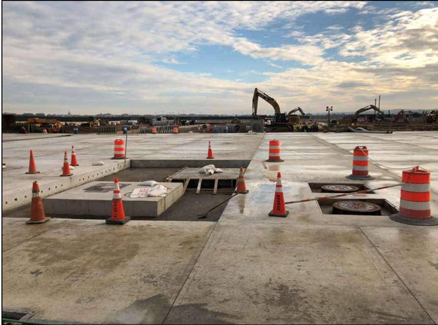
Apron Pavement – Outside Surcharge Completion: March 2019
