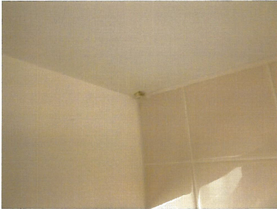
19. Non-ACM gypsum ceiling board with joint compound (DJ2-Samples 50, 51) in Restroom 171.01.
