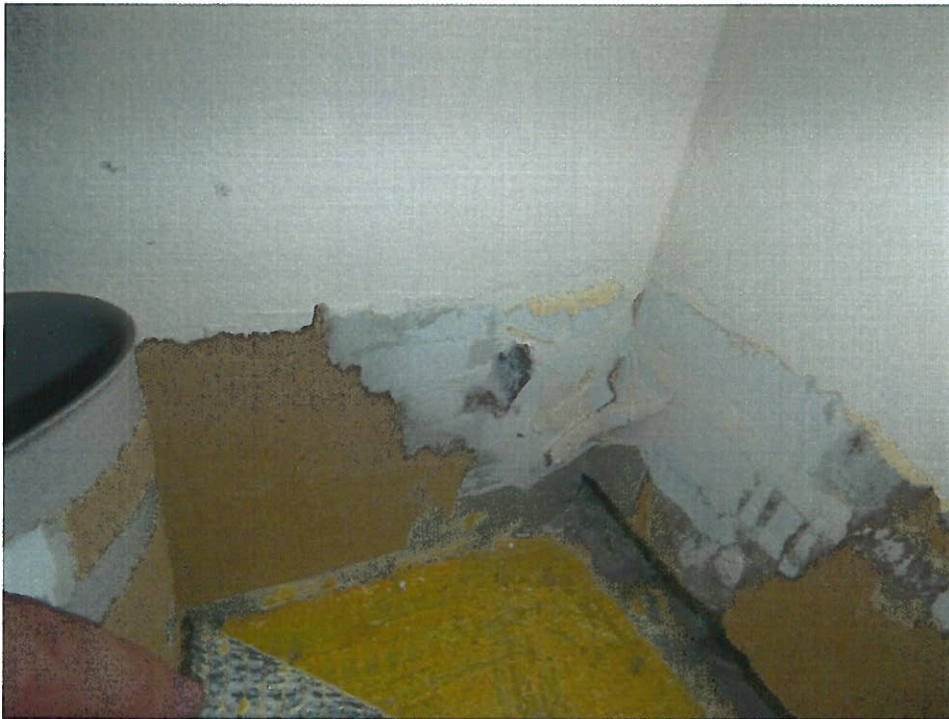
44. Non-ACM gypsum wall board with joint compound (DJ7-samples 153, 154) in Office 310.
