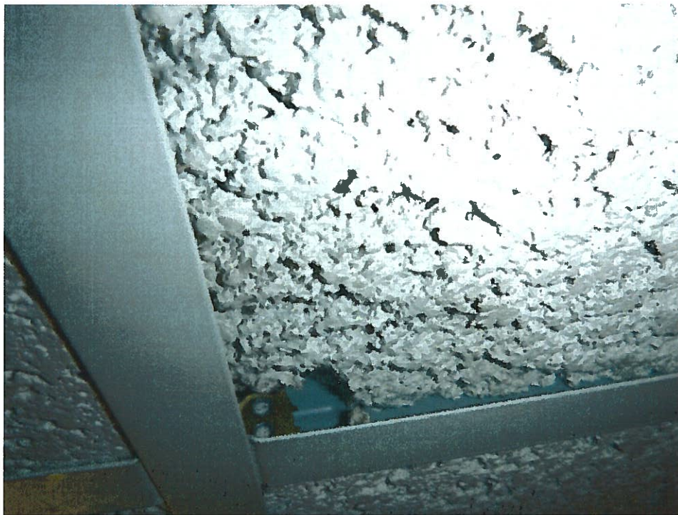
10. Non-ACM 2' x 2' heavy textured ceiling tile (CT1-Samples 23, 24, 104, 105) in hall outside Office 180.18.
