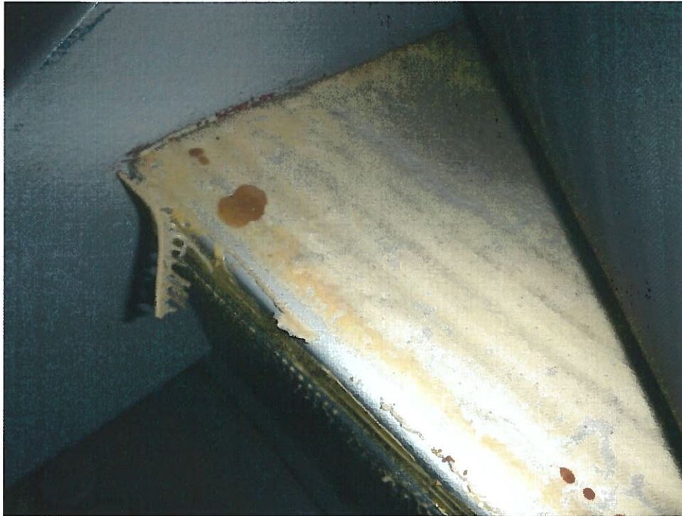
29. Non-ACM beige mastic on stair tread (STR1-Samples 96, 97) in Stair 1.
