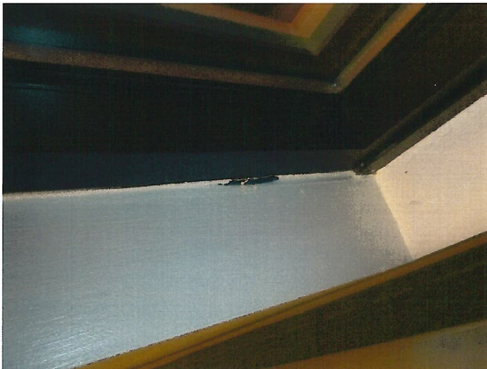
42. Non-ACM interior window caulking (CK8-Samples 149, 150) in 225.00 Bridge to hangar.
