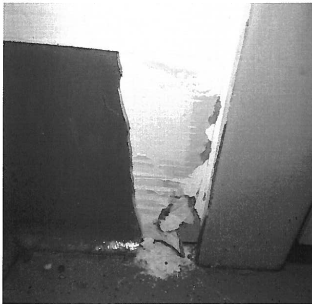
22. Non-ACM gypsum wall board with joint compound (DJ3-Samples 70, 71, 76, 119) in Rooms 101-112 and 201-221.
