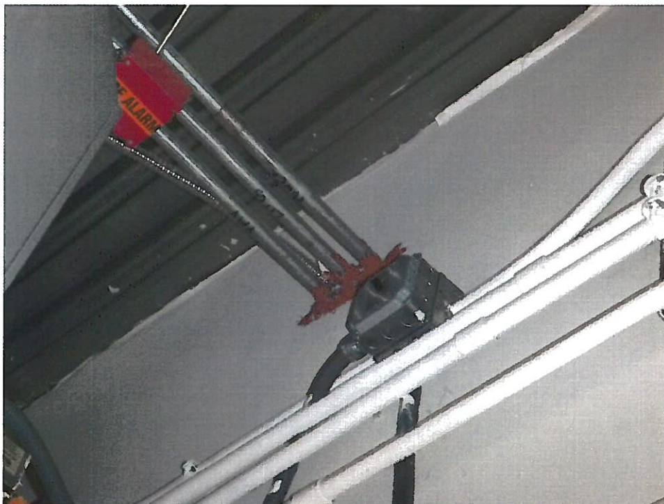
16. Non-ACM red fire stop (FS1-Samples 43, 44, 45) in Electrical Room 263.03.
