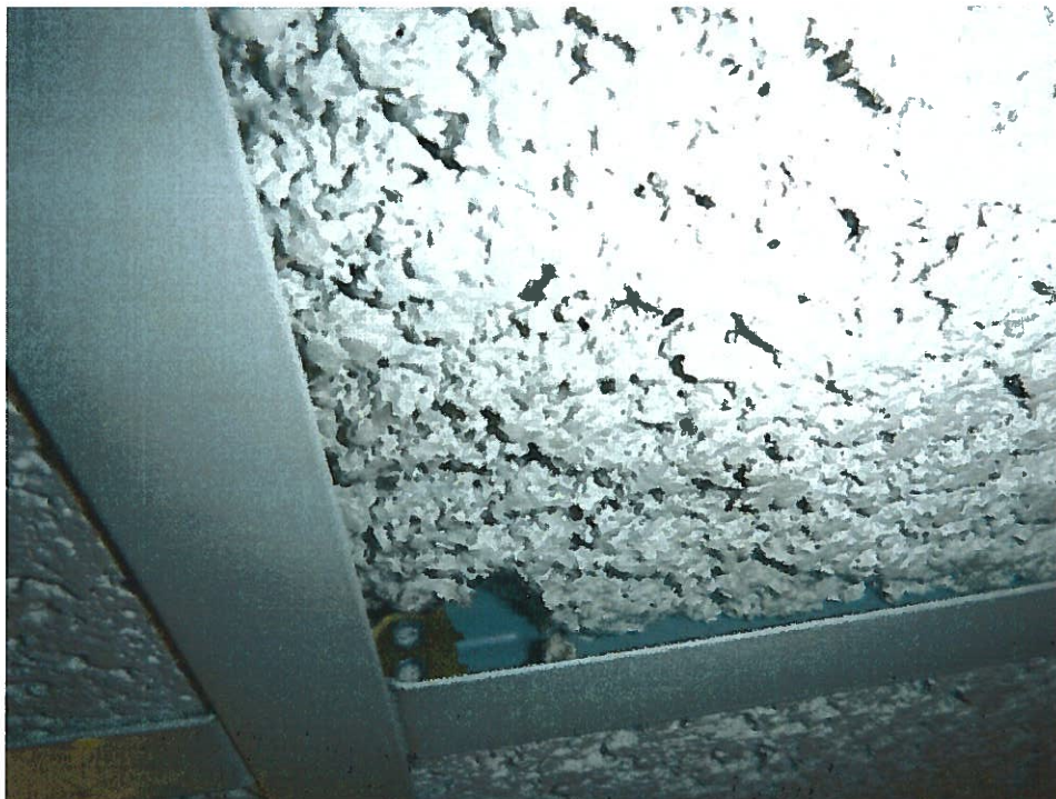
10. Non-ACM 2' x 2' heavy textured ceiling tile (CT1-Samples 23, 24, 104, 105) in hall outside Office 180.18.
