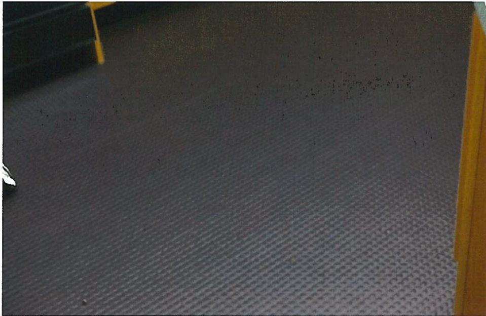
45. Non-ACM shiny maroon small square resilient sheet flooring (LN1-Samples 155, 156) in Room 311.
