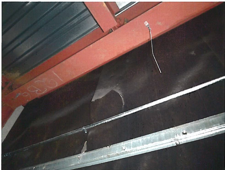
32. Non-ACM black felt paper on inner wall (WFL1-Samples 120, 121) in Reception 212.
