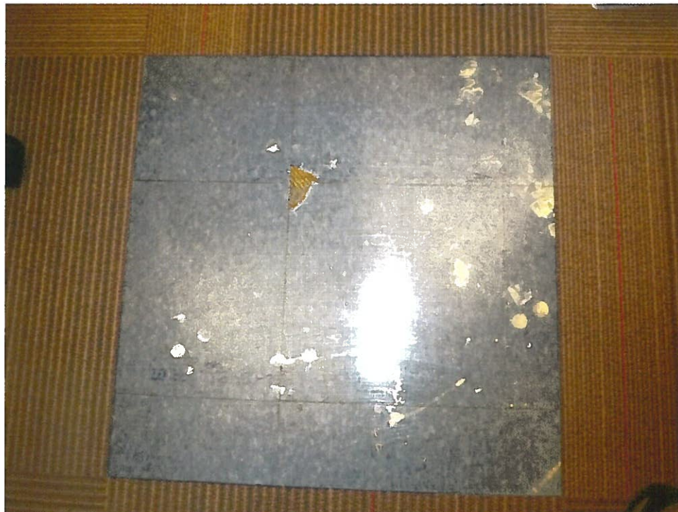
26. Non-ACM 12" x 12" dark blue with light blue feather floor tile (FT7-Samples 84, 85) with non-ACM yellow mastic (FM7-Samples 86, 87) beneath the floor tile in Room 138.39.
