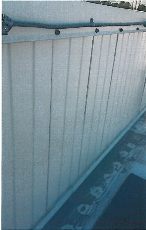
49. Non-ACM white caulking at roof perimeter (RCK1-Samples 163, 164) on exterior roof of building.
