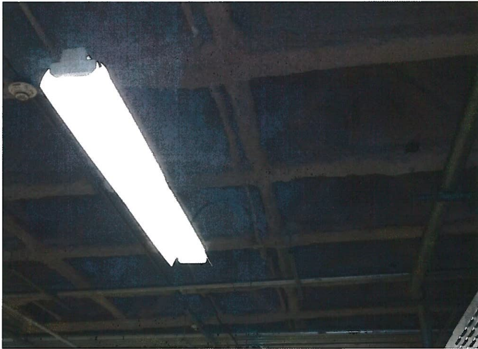
25. Non-ACM spray-on fireproofing on concrete ceiling deck (FP3-Samples 77, 78, 79, 80, 81, 82, 83) in Vault 100.
