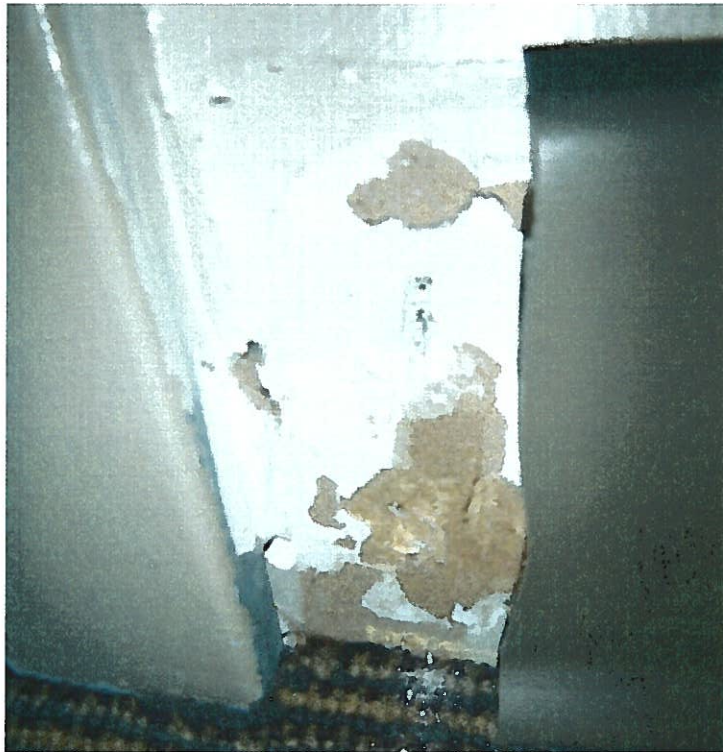
30. Non-ACM gypsum wall board with joint compound (DJ5-Samples 108, 109) in Conference Room 206.10.
