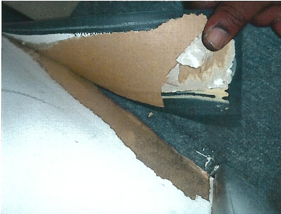
14. Non-ACM beige mastic on baseboard (BM1-Samples 34, 35) in Office 174.01.
