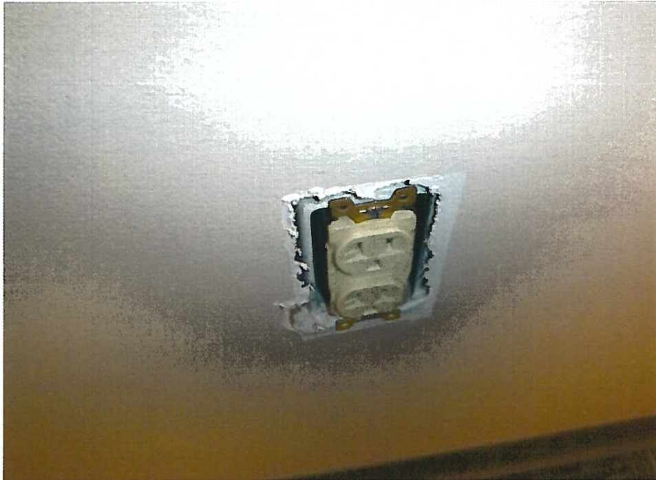
17. Non-ACM gypsum wall board with joint compound (DJ1-Samples 46, 47, 98) in Office 190.23.
