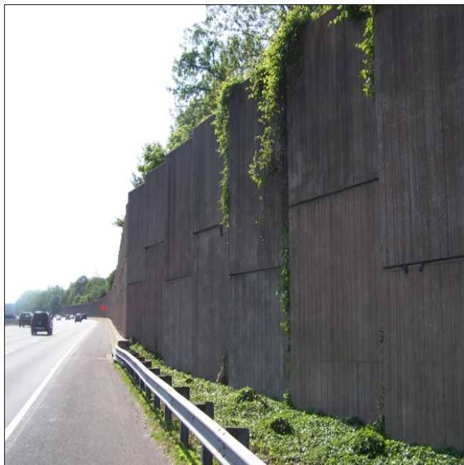
Existing Sound Walls
