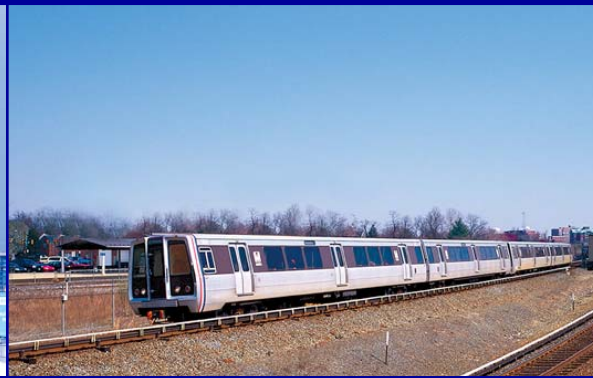
Dulles Corridor Metrorail Project
