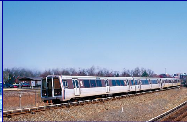
Dulles Corridor Metrorail Project
