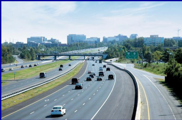
Dulles Toll Road
